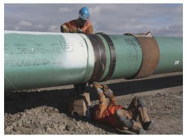
Pipeliners buffing the pipe following welding; more than 46,000 pieces of pipe were welded together to make one continuous pipe on our L3RP between Hardisty, Alberta and Gretna, Manitoba, which began commercial service in December 2019.
